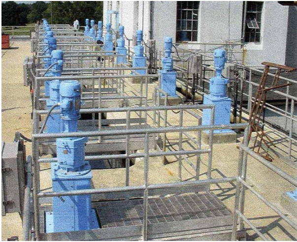
Series 1000 on flocculator duty - USA
