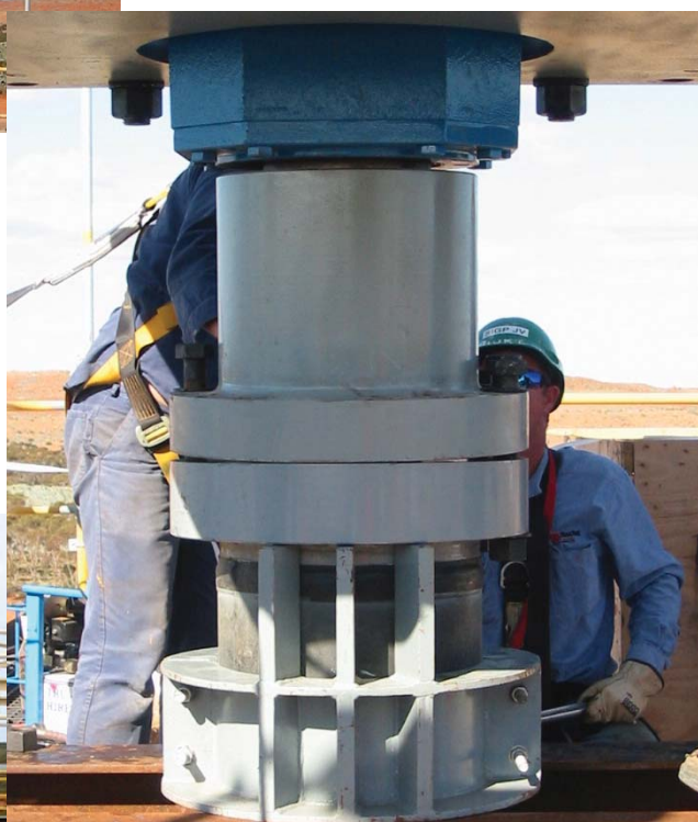
Mixtec Agitator shaft coupling and support collar
