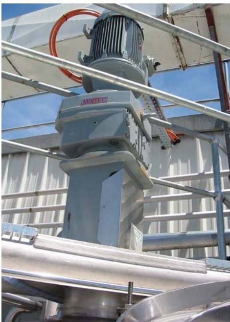
Series 2000 agitator on a crystalliser duty
